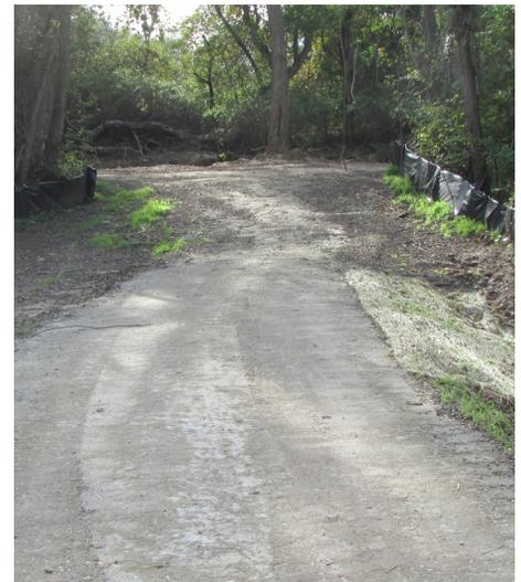
Raised road with aggregate directly on top of the wetland area
