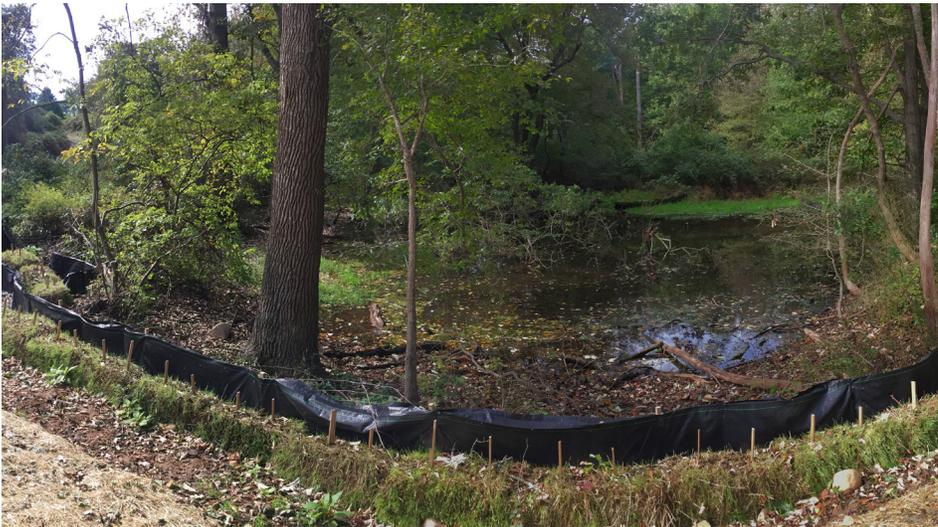
Heavy rains breached the fence depositing silt in pond. Photo by Caleb Lamont.
